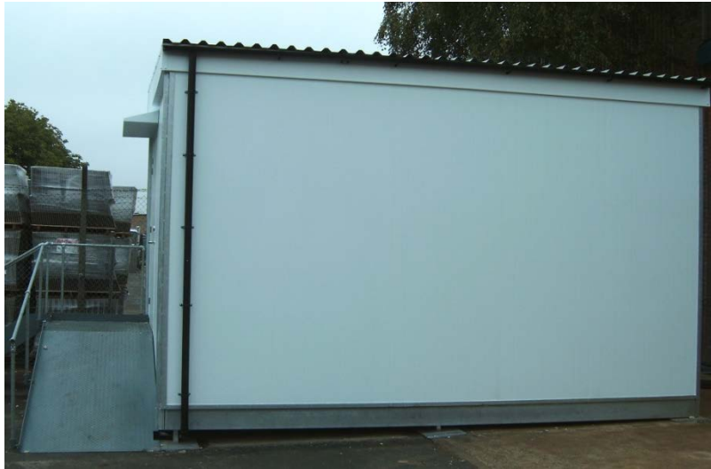
Small pods built on site
