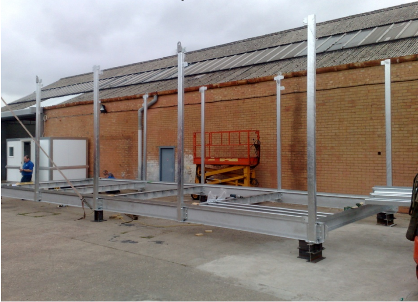
Prefabricated at factory and craned onto site
