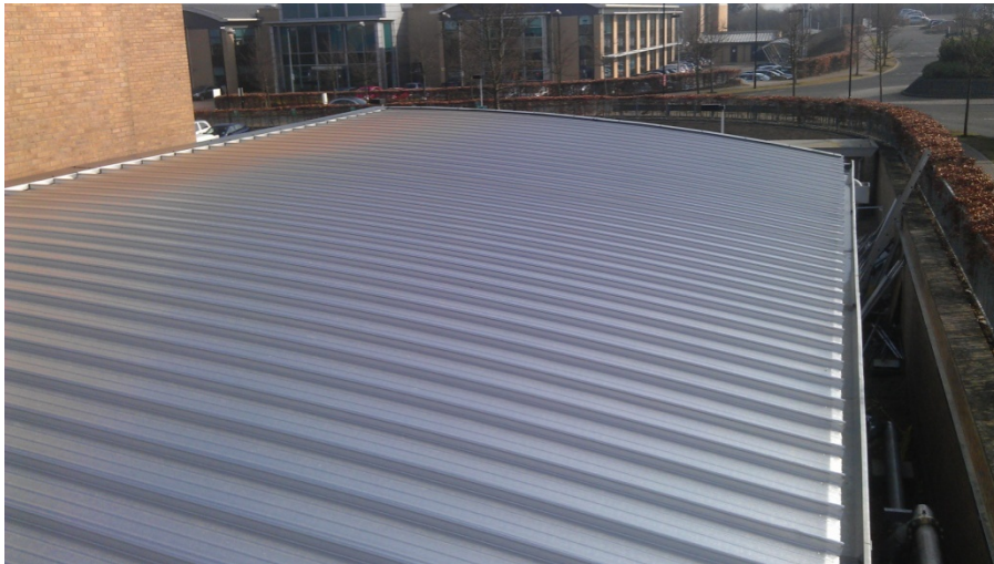
Curved roof with standing seam trays plus Kingspan cladding
